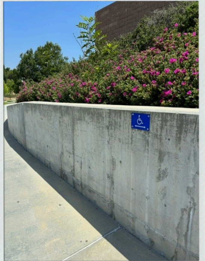
Walkway between The AC building and the AA building
