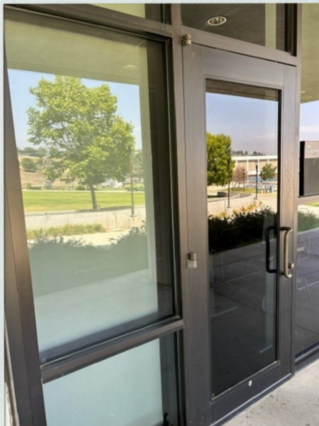
Classroom doors or windows
